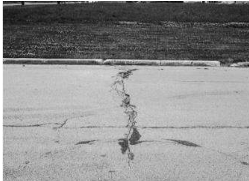
Figure 2-6: Example of Transverse Crack (ASTM)
