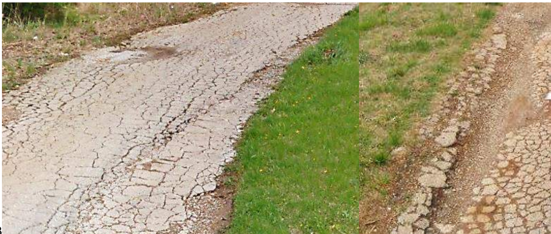
Figure 3-6: Insufficient Pavement Thickness
