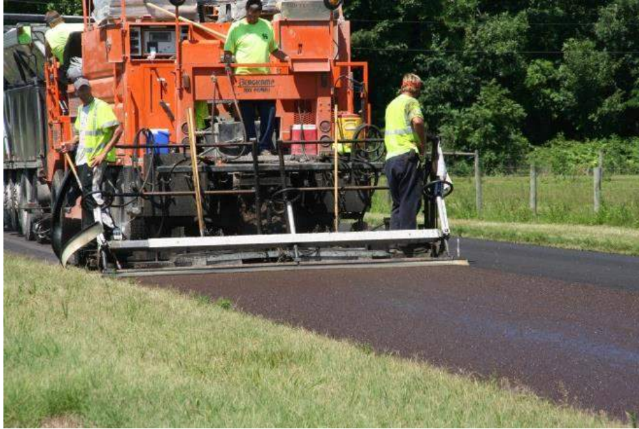
Figure 2-23: Microsurfacing Crew at Work. (Eric Pulley).
