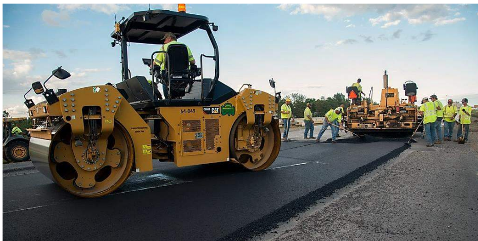
Figure 2-19: Reconstruction of I-94 (NDDOT)
