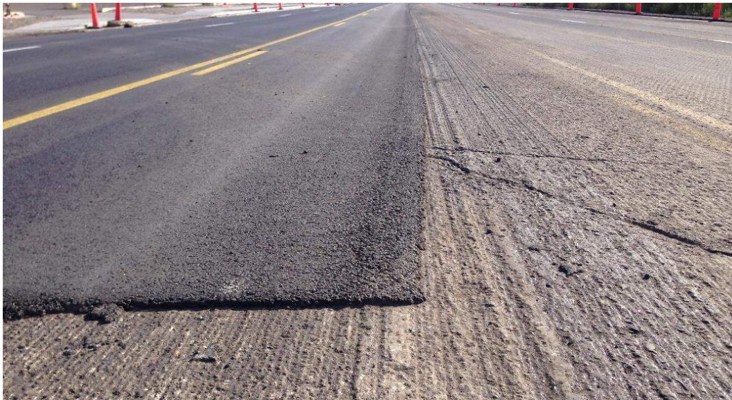
Figure 2-20: HMA Overlay Placed On Milled Pavement (Famartin)
