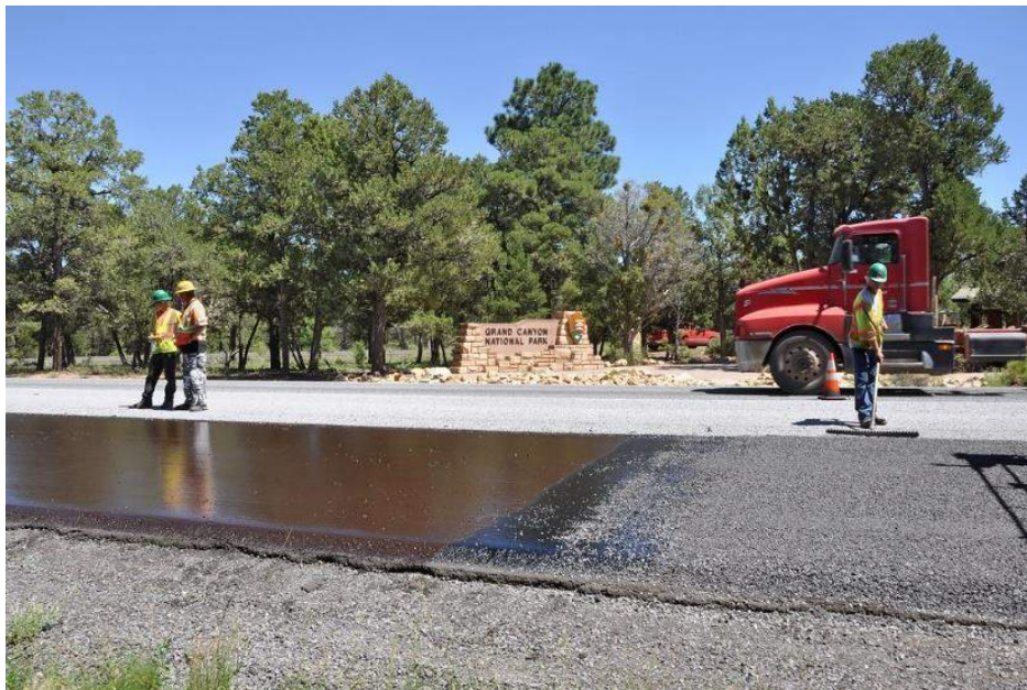
Figure 2-24: Cape Seal (Michael Quinn-NPS)
