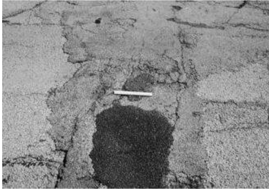
Figure 2-7: Example of Patching (ASTM)
