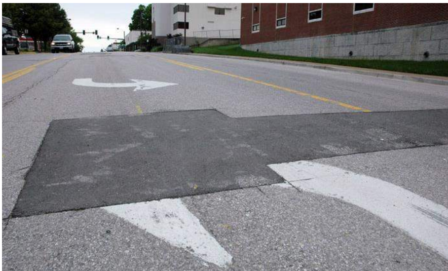
Figure 2-27: HMA Patching with Localized Pavement Removal (KOMU)
