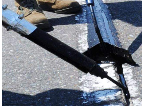
Figure 2-26: Crack Sealing Performed W/ Routing (USAF/Kenna Jackson)
