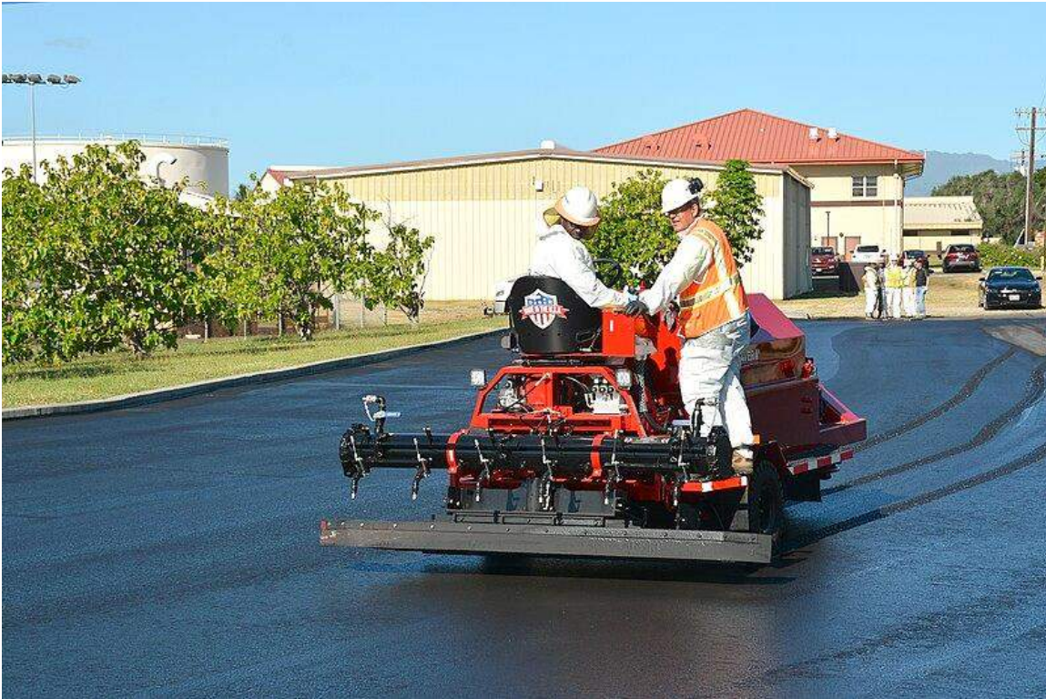
Figure 2-22: Slurry Seal Being Placed (NAVFAC)
